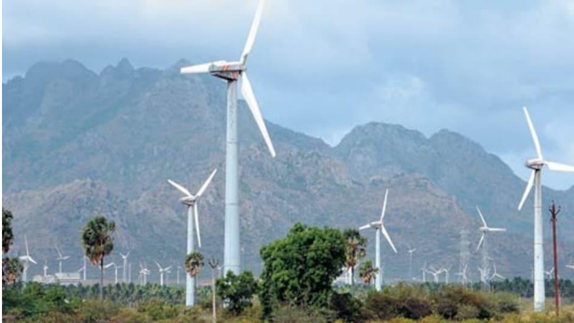
Fig.4. Muppandal wind farm
