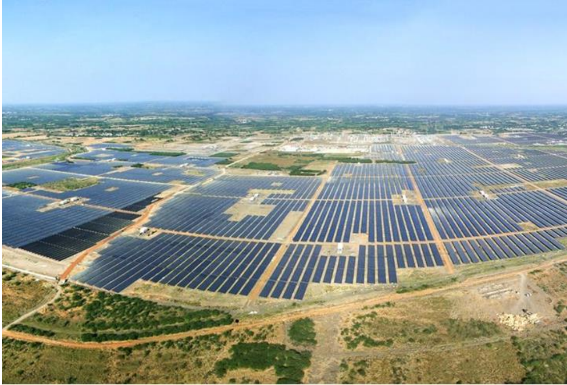
Fig.5. Solar plant at Kamudhi
