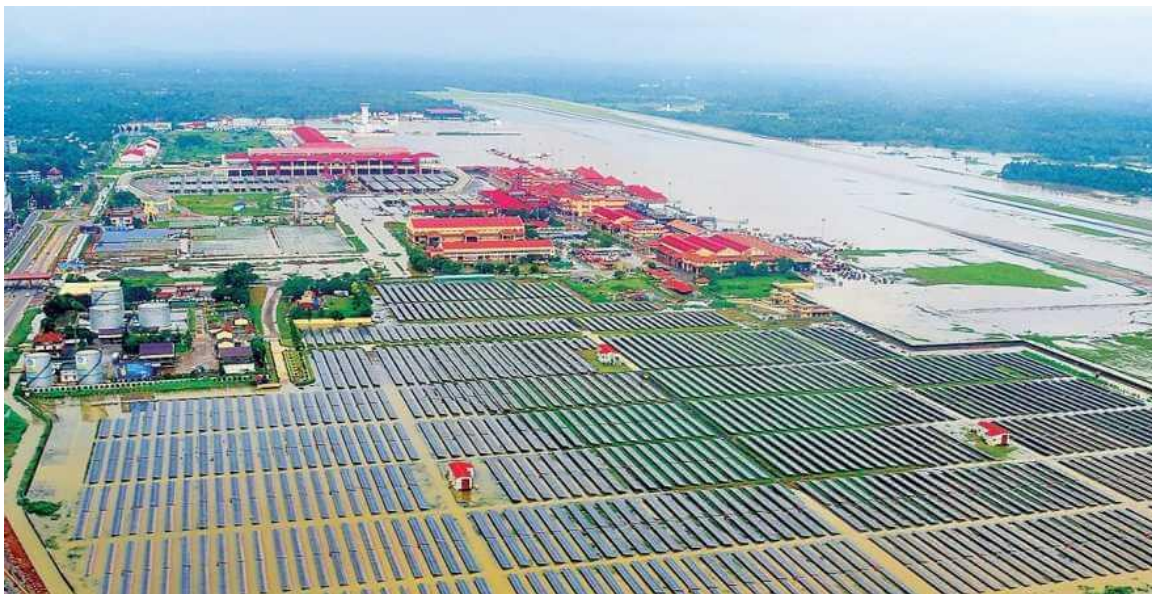
Fig.6 Solar plant at Kochi
