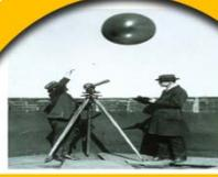
**1930:** Pilot Balloon Observations were taken for Wind Data measurements.
