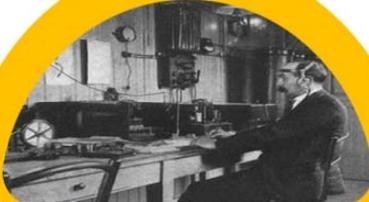
**1929:**With the installation of shortwave wireless by the Director General, Post & Telegraph at the Karachi civil W/T station, wireless sharing of synoptic weather data was possible.
