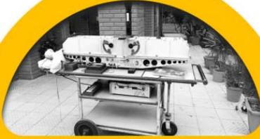
**1987:** First total column ozone measured by Dobson ozone spectrophotometer at Dakshin Gangotri, Antarctica.
