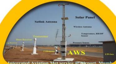
**2020:** Integrated Automatic Weather Observing System (AWOS) installed at major airport.
