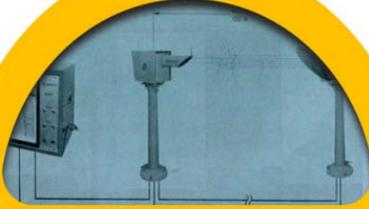
**1966:** At Dum Dum airport (Calcutta) was installed Transmissometer to assess the runway visual range (RVR).
