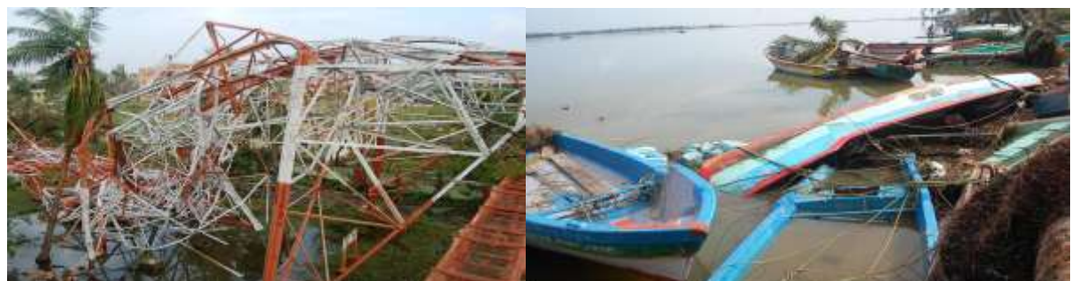
Fig. 2.2.8 Some damage photograph due to the cyclone THANE in Cudallore district Puducherry.
