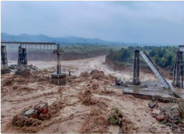
Collapsed portion of railway bridge over the Chakki river after flash flood triggered by heavy monsoon rains.(PTI)
